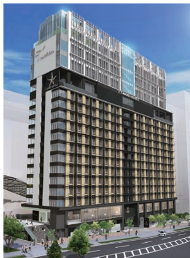
Universal City Station Project
