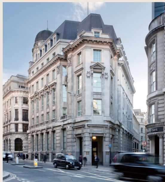
1 King William Street, the second office building we acquired in London, U.K.
