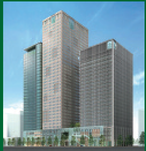
Otemachi 1-Chome Urban Area Redevelopment Project Type 1
