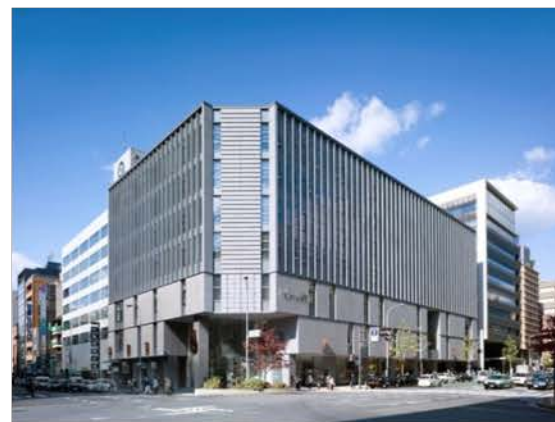
Urbannet Shijo-Karasuma Building (Completed in October 2010)
